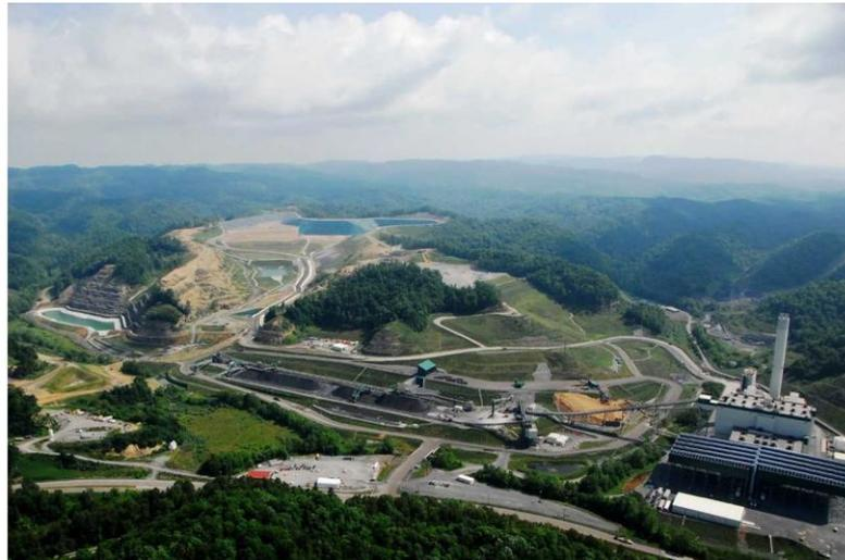
**The 600 MW Virginia City Hybrid Energy Center, USA, where two CFBC units fire waste coal and biomass (photograph courtesy of Dominion Energy)**
